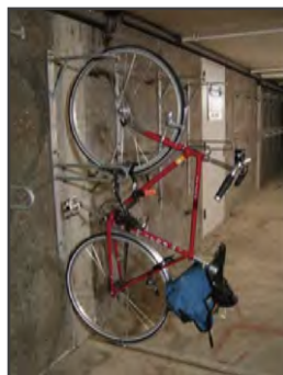
Figure 10: Vertical Bike Rack Dimensions are 2' wide and 6'4" tall. Racks should be distanced 24" from each other.
