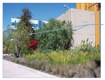
A variety of shade trees are used on the south facade for passive cooling
