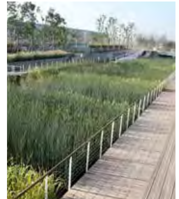
Constructed wetlands treat wastewater {Shanghai, China}
