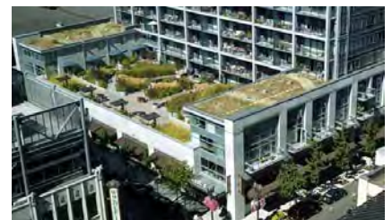
Example of a green roof.
