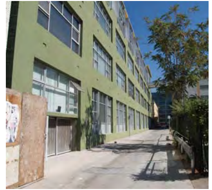
Residential units are not permitted on the ground floor adjacent to non-pedestrian priority alleys as shown here.
