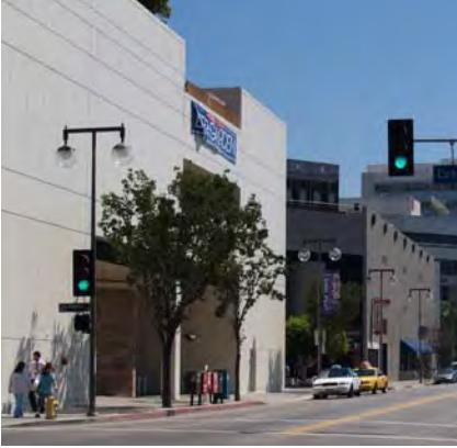
Bad example of building façades that provides little to no visual relief and too much blank surface.
