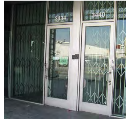
Interior grilles that are more than 75% open are less visible during non-business hours and easier to screen from view during business hours.
