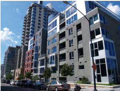
6- and 7-story street wall
