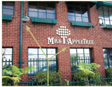
✓ Simple and straightforward signs, using quality individually cut letters with gooseneck lighting fixtures for direct illumination
