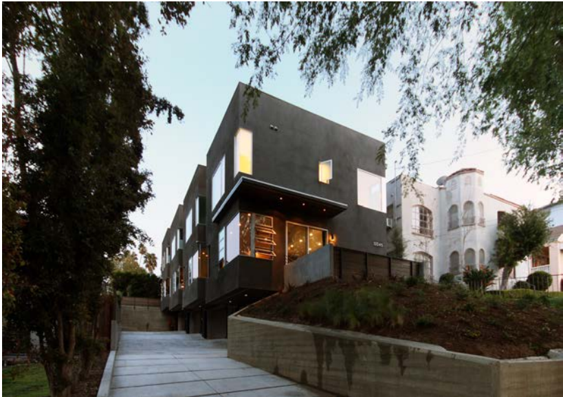
The slightly sloping site resulted in the units having a “stacked” configuration and the garages being cut into the slope. A 35 foot front setback was provided
