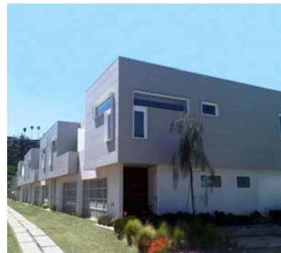
Rock Row uses permeable paving to provide a more hospitable pedestrian path along the driveway.
