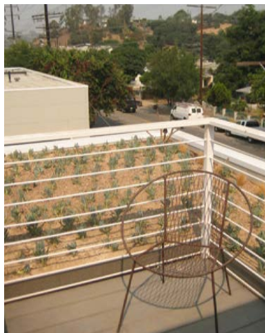
A green roof helps absorb runoff, reduces the heat island effect, and provides an attractive amenity for residents.
