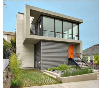
A permeable driveway (concrete grid filled with grass) increases storm water infiltration on the small lot.
