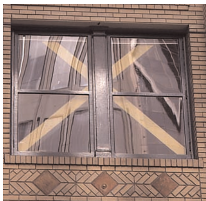
This unreinforced masonry building was structurally upgraded using steel X-bracing. This type of system is often visible from the exterior through windows; care should be taken to design these systems with the least visual impact.
