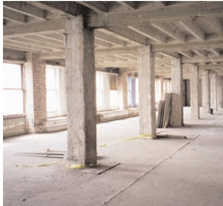
The column grid and the typical windows at the Broadway and Spring Street elevations. The grid could remain exposed in either an office or residential reuse scenario.
