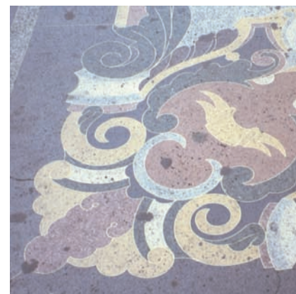
A detail of the terrazzo outside the Los Angeles Theater. The accumulation of gum is evident on the surface.
