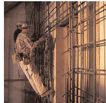
Shotcrete, spray-applied reinforced concrete, is another method of seismic strengthening.
