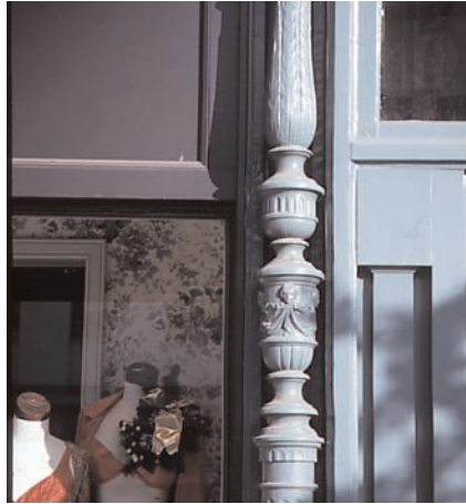
Historic structural elements such as this cast iron column should be retained.
