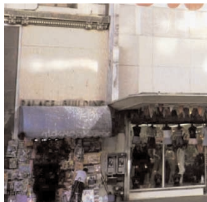
The main building entrances at either side of the Palace Theater are presently not evident due to the existing facade application. The above image shows a storefront located within one of the original openings.
