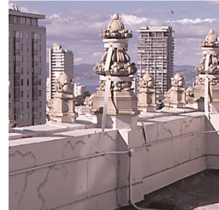
Stabilization of roof top ornamental elements should be undertaken immediately to ensure safety of pedestrians below.
