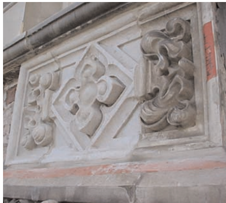
An example of replacement terra cotta elements. Cracking and spalling are common signs of water infiltration with terra cotta. The metal attachments become deteriorated and damage the terra cotta.
