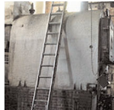
Historic buildings commonly were heated with a boiler and steam heat. These types of systems often must be upgraded during rehabilitation.
