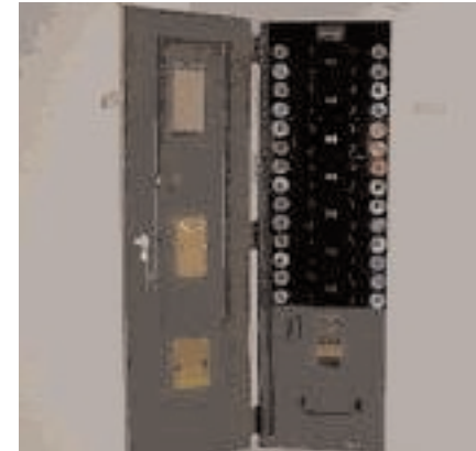
Older electrical service can be a hazard. Note the old fuse system in this photograph. A modern circuit breaker system will likely need to be installed in this building.
