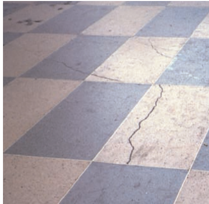
A detail of a cracked terrazzo sidewalk within the study area. While some terrazzo is highly decorative, other elements are composed of simple repetitive patterns.
