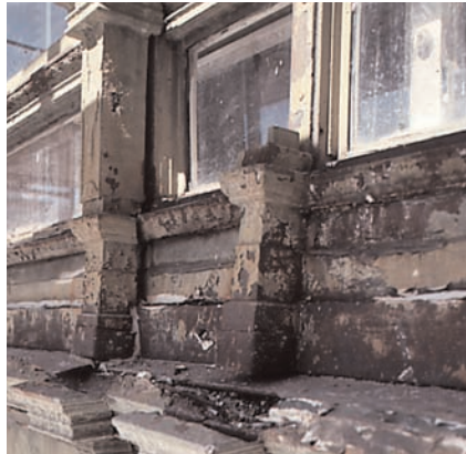
Deteriorated exterior painted surfaces frequently contain lead, which should be professionally abated.
