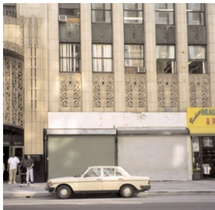
Roll down doors are one of the major intrusions within the study area. These features cover and detract from the historic components of storefronts.
