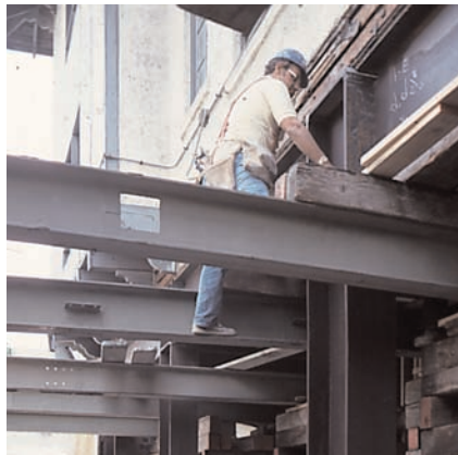
Any unstable condition should be temporarily shored, with minimum damage to the historic building.
