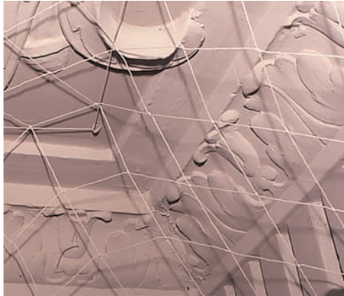
This nylon mesh system provides temporary protection from falling plaster until rehabilitation can be undertaken.
