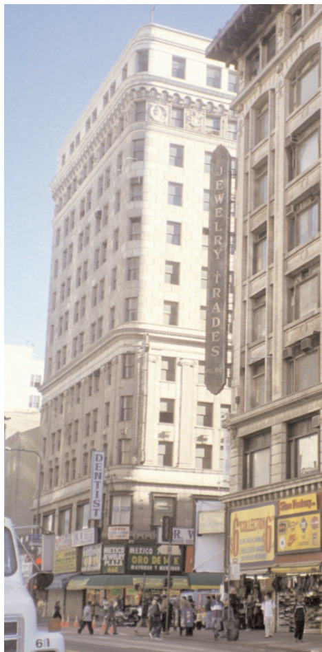
This corner building is a classic three-part commercial building consisting of the base, middle, and top. A phased approach to rehabilitation of this structure could start with the storefronts, then move to the upper stories, including terra cotta and window survey and then repair, if necessary.
