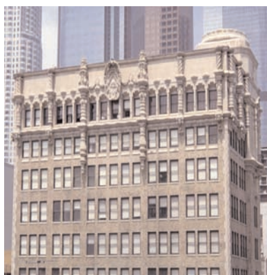
Replace in Kind: The upper story windows at the Million Dollar Theater are good examples of new features that replaced older windows with a similar type and style of window.
