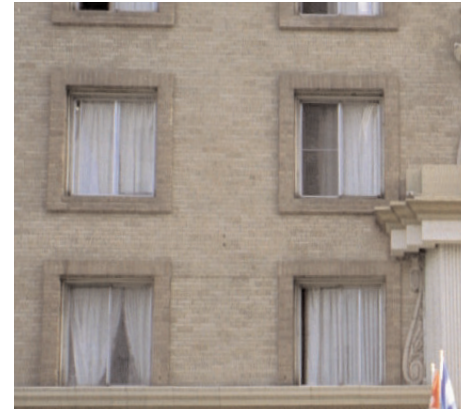
These replacement aluminum windows do not provide the same sense of detail or scale to the building facade as the originals. The lack of window mullions disturbs the facade proportions.
