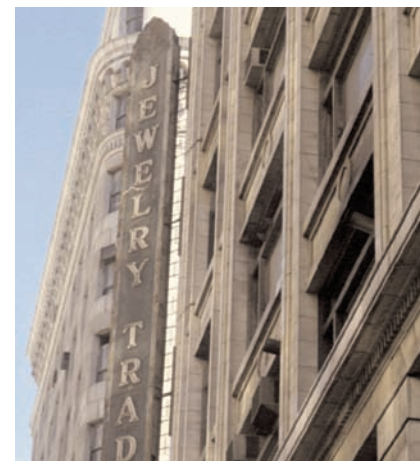
The Jewelry Trades building sign is metal and it is anchored to the building with metal ties into the terra cotta.
