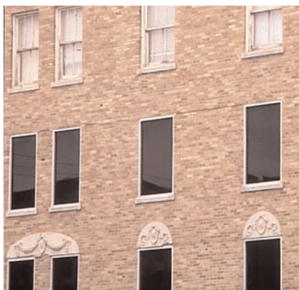
A detail of the original windows above and the replacement windows below.
