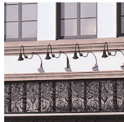
These goose neck exterior wall-mounted fixtures cast light down onto the store's display glass and sign area.
