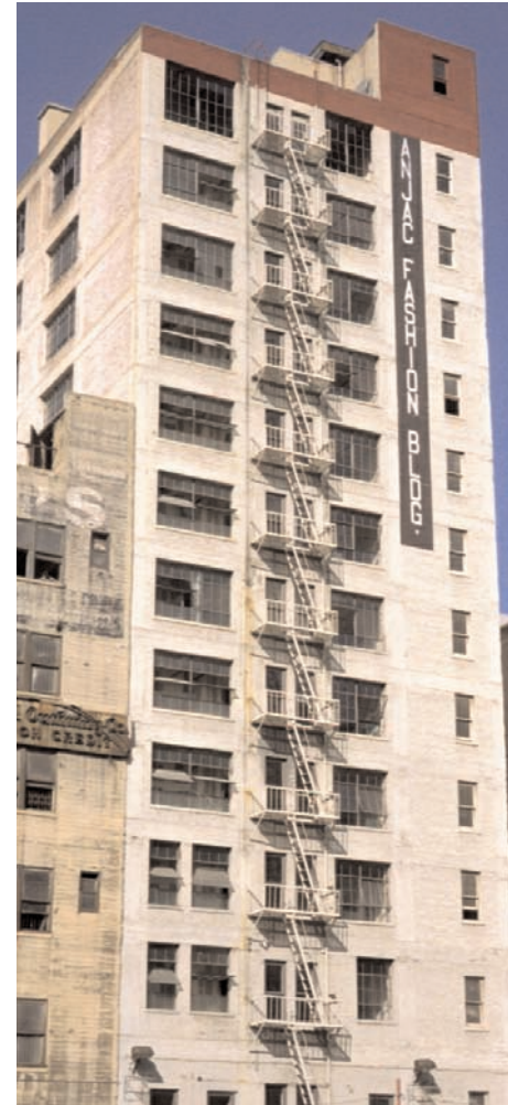
Rear facade materials and features include brick, painted signage, punched openings, fire escapes, and industrial sash windows.
