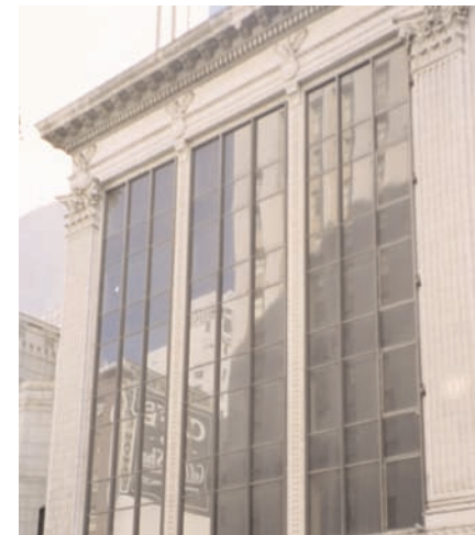
This building has tinted replacement windows that diminish the intended lightweight nature of the structure.
