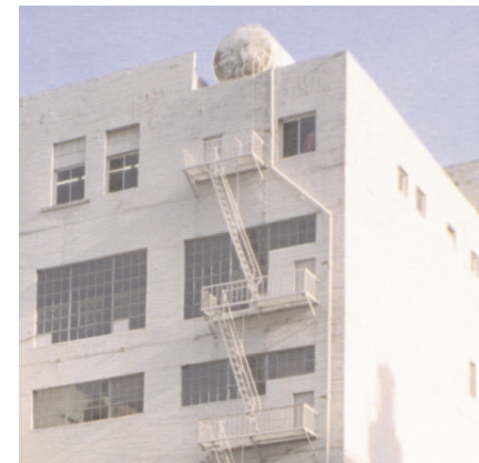
This roof has a large tank visible from the alley behind the building. Tanks of this sort should be checked for hazardous materials. If these elements are obsolete and are not character-defining features they should be removed.
